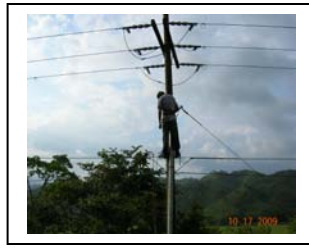
Tapping into high voltage lines
