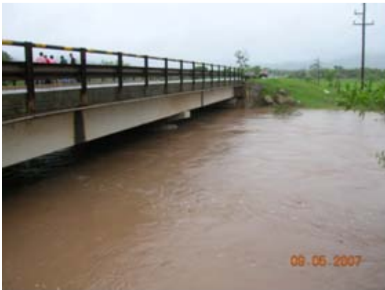
The swollen Jagua River after 24 hours of rainfall
